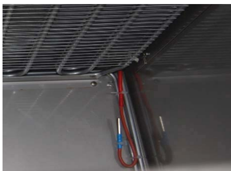
Mounting of the sensor in the freezer
