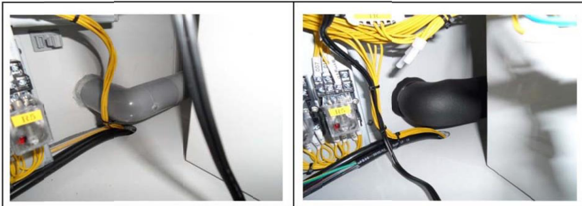
Assembly of Main Frame of Exhaust Pipe-A
