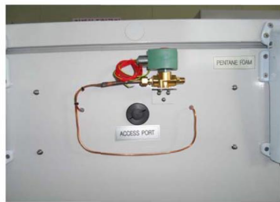
S/V+Capillary Ass'y-B
