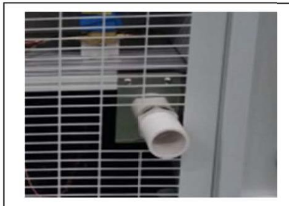
Work of Packing of Protruding Part of Exhaust Pipe-C
