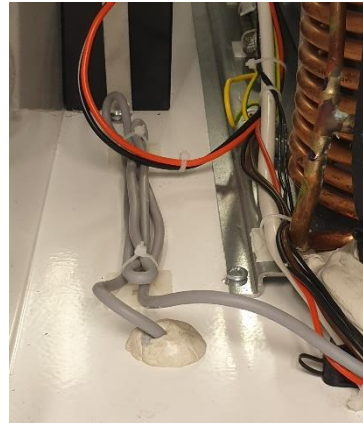
Introduction of the sensor from the top of the engine compartment
