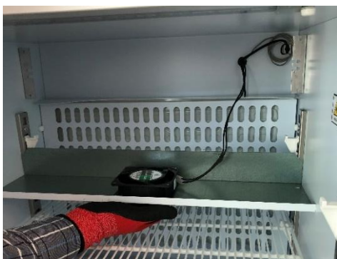
3-Remove fan protection, unplug fan and plug new one
