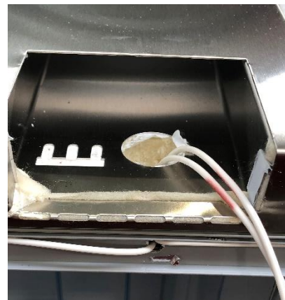
4- Disconnect, remove the heater and change for new one
