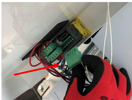
3- Probe is connected in the controller
