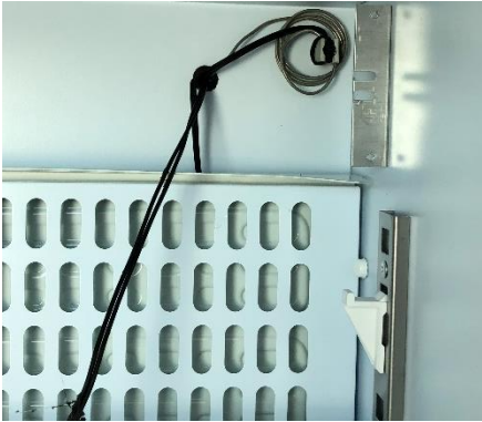
1-Remove cover and screws of evaporator protection
