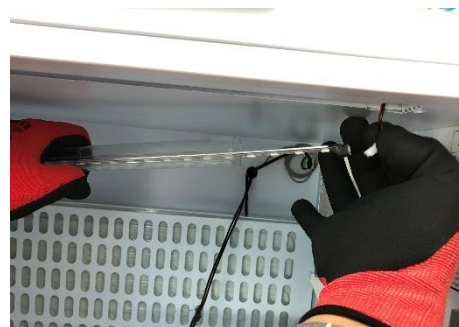
4-Unplug led strip and change for new one
