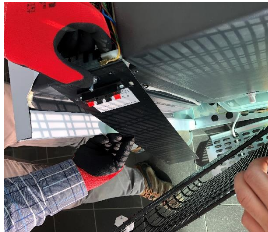
5- remove black metal protection to access hole for cables inside unit
